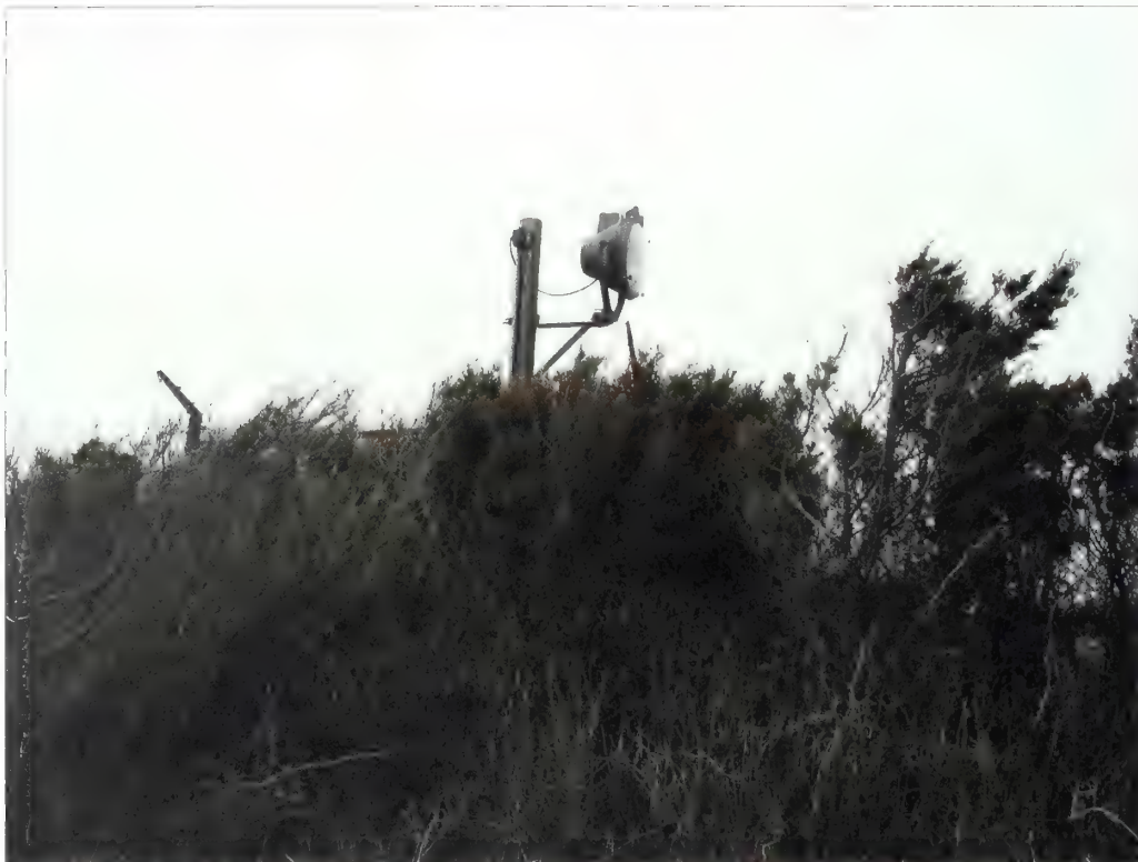
Figure 3.71. Floodlight, NIKE launch site. At the Missile Magazine area, eight floodlights are positioned along the inner fence. Each light features a parabolic fixture mounted with a metal bracket to a wood pole. Six similar lights are located at the Missile Maintenance Area on the engineered earthworks (Olmsted Center, April 2008).
